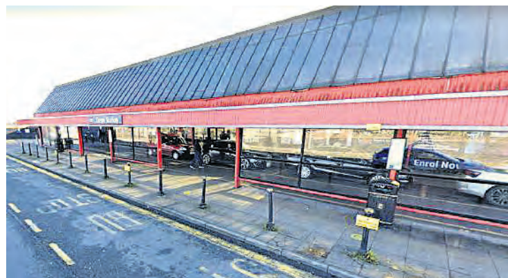
Crewe railway station
